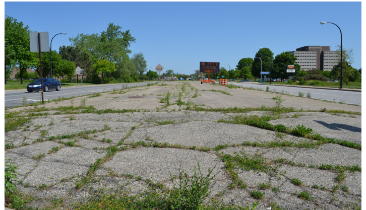
Concrete medians dominate the landscape in Area 2
