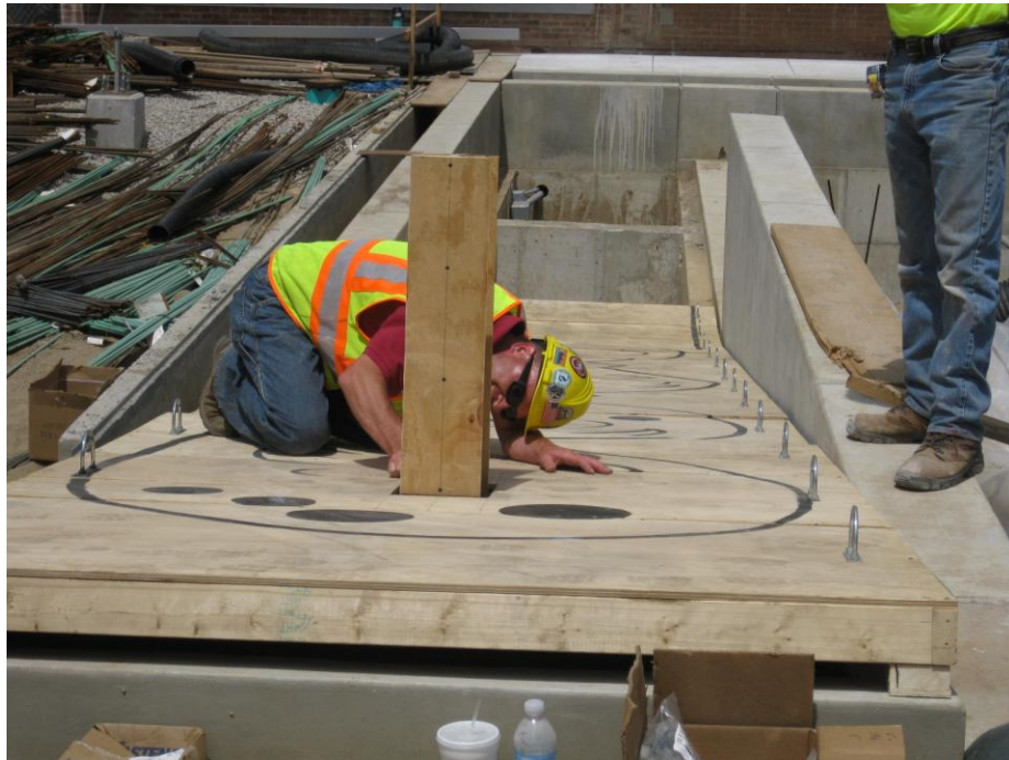
Marking elevations of ramp templates on structure mock-up
