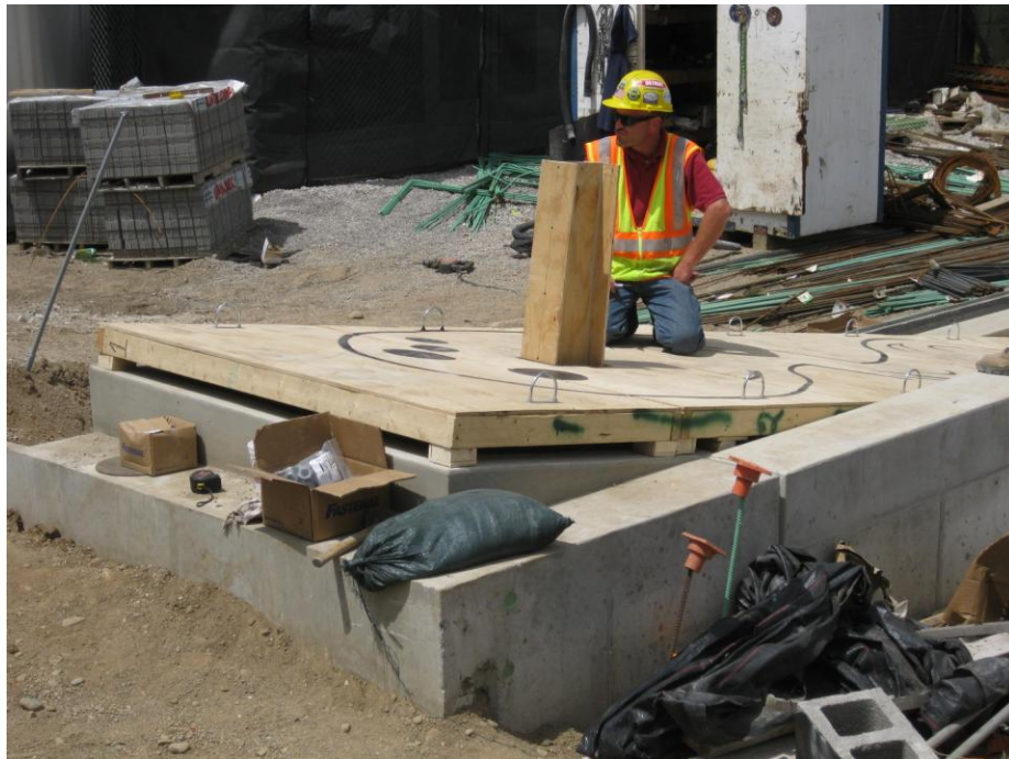
Templates in place, showing position of ramp and structure.
