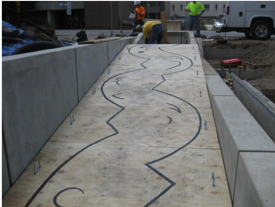
Plywood templates being "fitted" on site. The black lines show the flow-way that will be formed in the precast concrete ramp.
