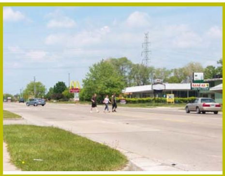
Inadequate pedestrian crossings
