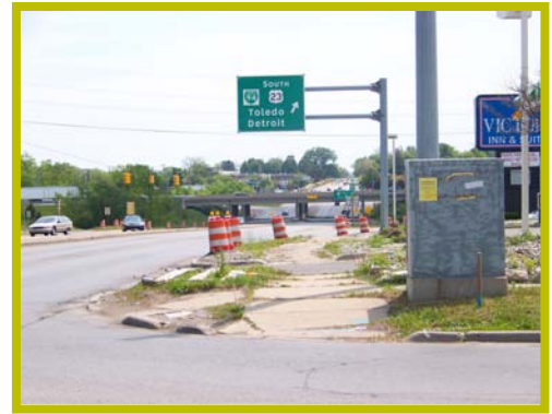
Intermittent and failing non-motorized infrastructure
