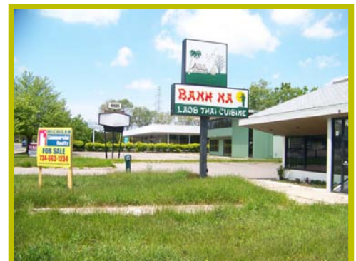
Numerous vacant parcels and high vacancy rates of commercial storefronts
