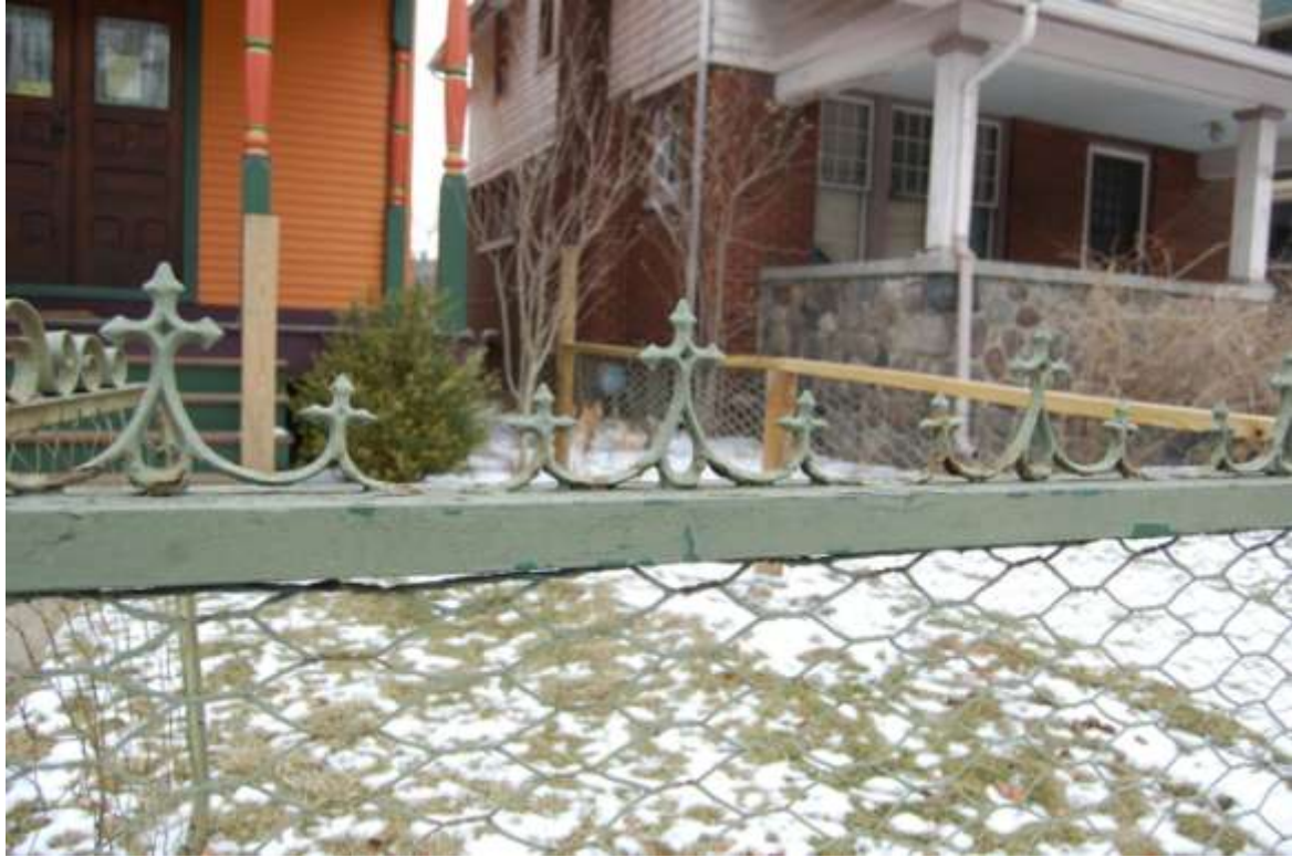
Photograph 13 – Detail of wood and wrought iron fence at 442 South Fourth Avenue, February 2010
