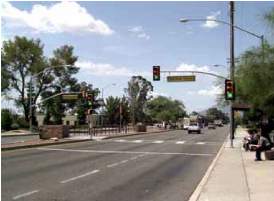
Figure 1-9: A picture of a midblock traffic signal.
