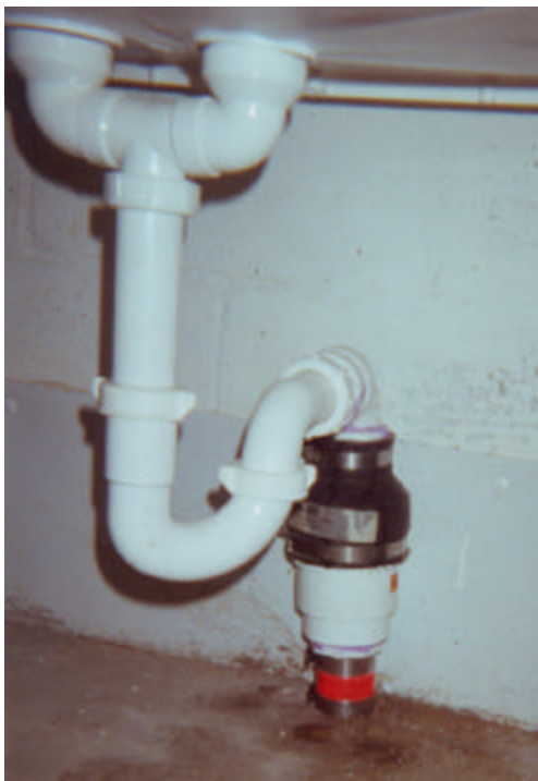
Figure E-10. Vertical Check Valve
