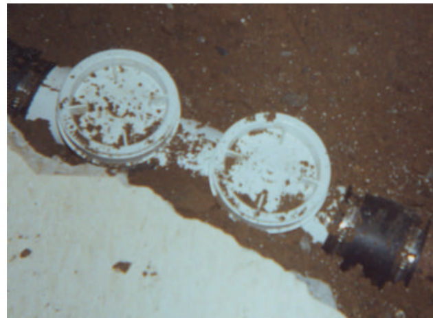
Figure E-11. Flap Check Valves
