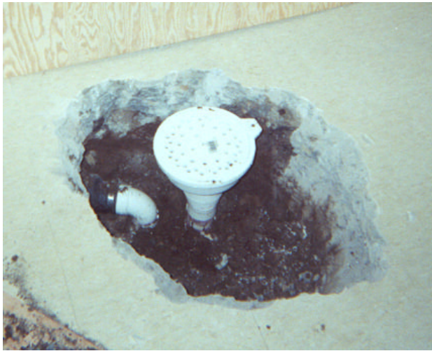
Figure E-9. Floor Drain
