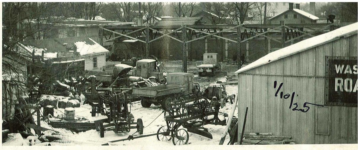
January 10, 1925 photo of the new Warren trusses on the garage going up in front of the old 12 bay garage. The existing concrete machine shop is visible on the left. As the new garage was being erected, most of the old garage with the exception of the one story wall fronting Washington Street was demolished and a new second story was added.
