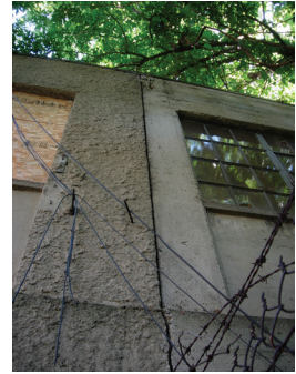
Photo with 1925 building (on left) and 1928 addition (on right). Stucco covers the earlier building, while the later addition was left uncovered.
