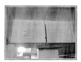
**C5 – Beam Delaminations:** There is some corrosion induced deterioration of the concrete beams in this structure. The deterioration is a result of ongoing corrosion.
