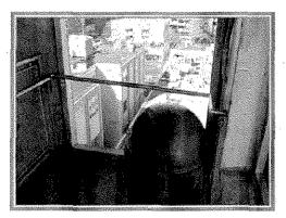
M2 – Handrail Repair: A hand rail in the North stair tower at Level 7 has been rotated out of place. This hand rail should be repaired to prevent possible pedestrian injury. Placement of an additional support at the right hand corner after the pipe railing has been reset will prevent this rotation from reoccurring.
