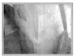
C3 – Column Delaminations: Columns and shear walls throughout the structure are in good shape overall. A majority of the column delaminations are located on Level 4 and consist mostly of failed patches. These locations should be repaired to prevent damage to the structural steel reinforcement in the columns.
