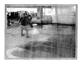
W7 – Sealer: A silane sealer was applied to all supported concrete areas during original construction in 1999 and then in 2007. Silane sealers help to reduce water and chloride intrusion into the concrete that may lead to corrosion of the embedded reinforcing steel and embedded connector plate steel over time.
