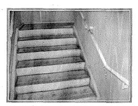
W6 - Deck Coating (at South Stair): Surface corrosion was noted on the steel in the South Stair. The corrosion is minor and has not created significant section loss. However, if no protective action is taken, the corrosion will become more severe and will eventually result in costly repairs. We recommend cleaning the steel to remove corrosion and deck coating the treads, risers and landings at the South Stair to protect the steel from further corrosion.
