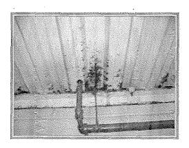
M1 – Clean & Paint Steel (at South Stair): As stated in Item W6, corrosion was noted on the steel in the South Stair. Corrosion was also noted on the handrails in the South Stair. In addition to deck coating the South Stair, as recommended in Item W6, we recommend cleaning the steel to remove corrosion and repainting the underside to protect against further corrosion. The handrails should also be repainted.
